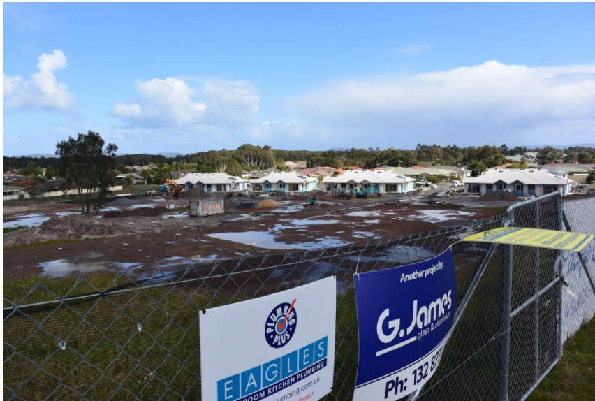
Figure 7: Pacific Cape villas under construction
