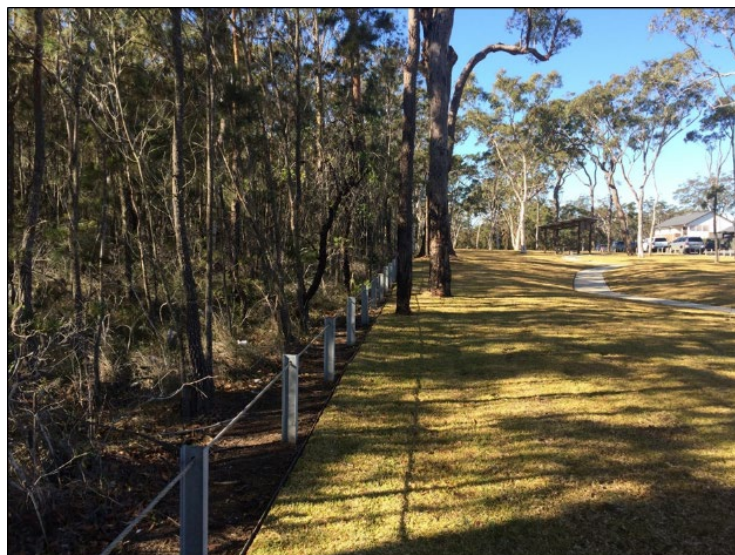
Figure 17: Example of bollards delineating cleared areas
