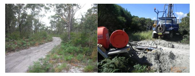
**Photo 1** on the left shows the sandy soils that are encountered throughout the development area. **Photo 2** on the right shows sand extracted during the development of production borehole LC 12-01 PB.
