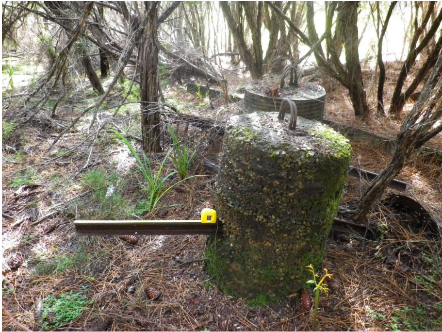
Plate 5 Concrete filled drums
