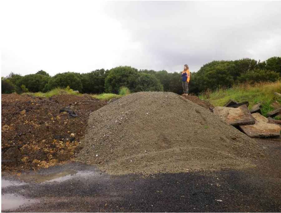
Plate 7 Material stockpile in general location of the Tuncurry-Forster Aeroclub site.
