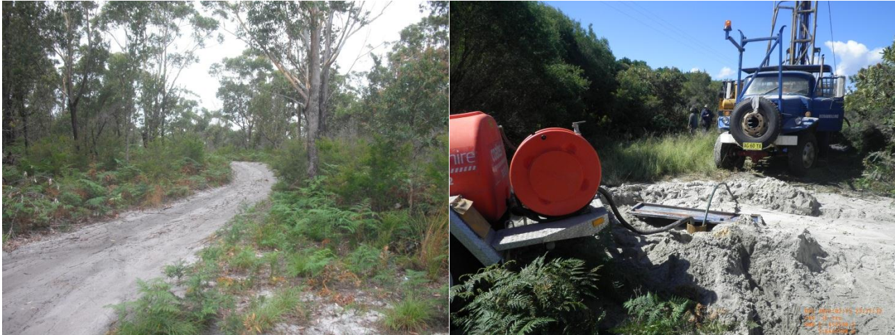
Photo 1 on the left shows the sandy soils that are encountered throughout the development area. Photo 2 on the right shows sand extracted during the development of production borehole LC 12-01 PB.
